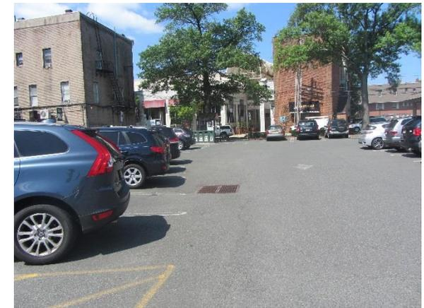
Parking spaces can be converted into pervious pavement to infiltrate parking lot runoff. A preliminary soil assessment suggests that more soil testing would be required before determining the soil's suitability for green infrastructure.
