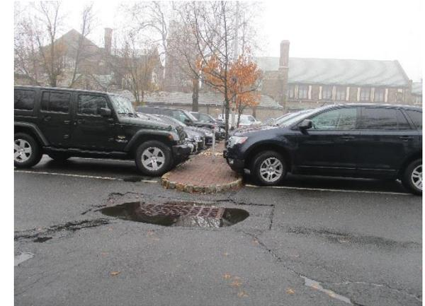
Parking spaces can be replaced with pervious pavement to infiltrate stormwater. A preliminary soil assessment suggests that more soil testing would be required before determining the soil's suitability for green infrastructure.
